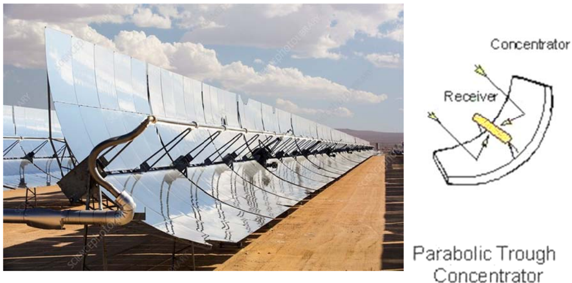
Figure 2 - A single-axis tracking parabolic trough collector.
